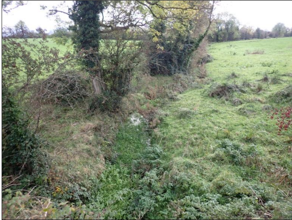
Plate 25 Heavy vegetation overgrowth encroaching on the watercourse at Site 22, upstream of Site 21 on the Lackelly East Stream.
