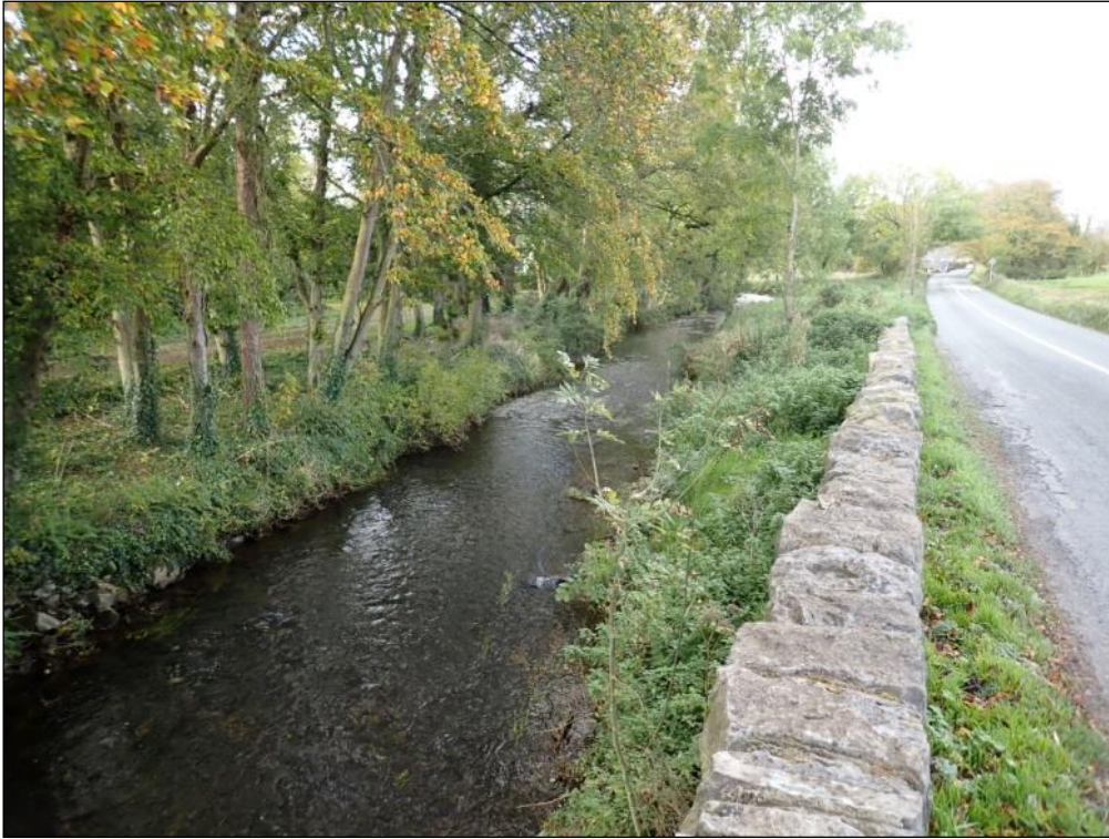
Plate 7 Site 7 on the main channel of the Drumcomoge, downstream of Knocklong.
