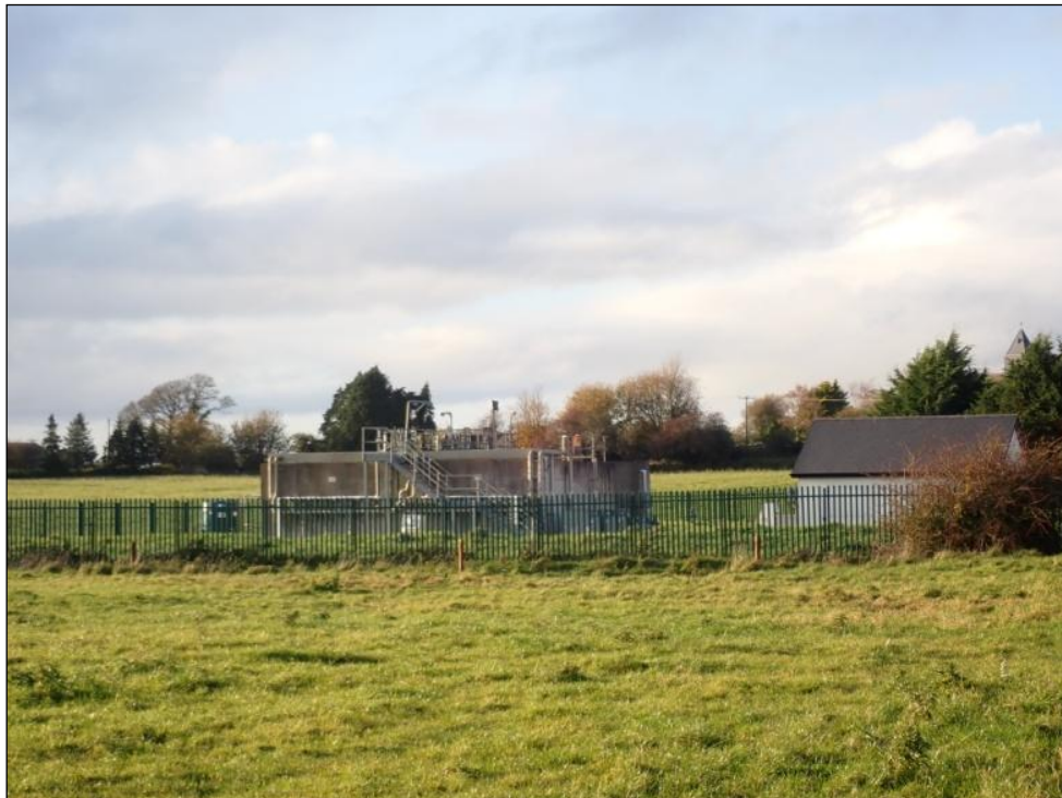
Plate 30 Emly Wastewater Treatment Facility which discharges into the Emly 24 near Site 26.
