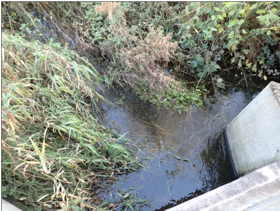
Plate 32 Water silted in the Emly 24 Tributary at Site 27 and encroached by vegetation from the banks.
